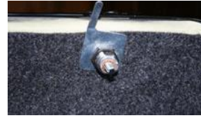
3. Replace lock into hole as this will act to locate liner into position.
