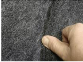
2. Flip over the liner and smooth out the seams.
